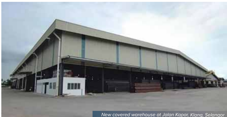
New covered warehouse at Jalan Kapar, Klang, Selangor
